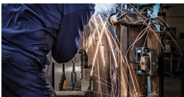
Welding of frame
